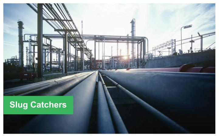
Large quantities of multiphase oil and gas flow in a pipeline often result in the formation of a much heavier, slow-moving fluid, known as Slug, with higher density compared to the main body of the flow. Effective separation of different impurities from oil and gas in upstream operations is a matter of paramount importance; since the efficiency of processing equipment and downstream activities is highly dependent on the purity level obtained at first stages.
