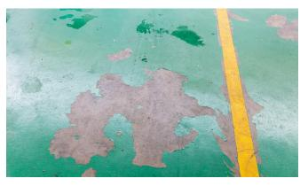
Polyurethane coatings are more resistant to diluted acids; so, the floorings will experience a degree of corrosion in extreme chemical environments. Furthermore, PU floorings are more likely to abrade and extremely sensitive to humidity which cause challenges in installation process.
