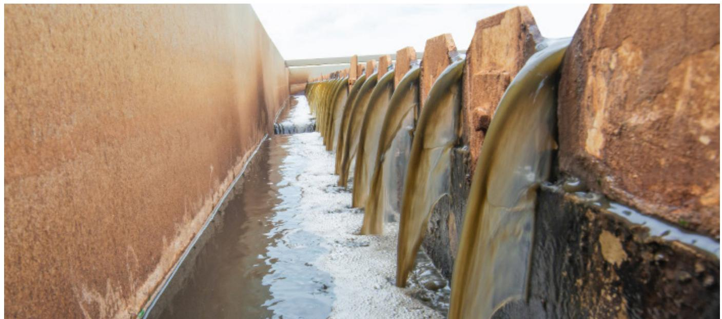
Corrosion affects different structures in contact with industrial wastewater and effluent streams, specifically the ones with continually varying liquid levels, such as ponds and storage areas, leaving damp surfaces exposed to sunlight and oxygen in open air. The presence of corrosive by-products, specifically hydrogen sulfide, would also gradually deteriorate surfaces made of concrete, iron, steel, etc., resulting in wall thickness loss and finally collapse of infrastructures.
