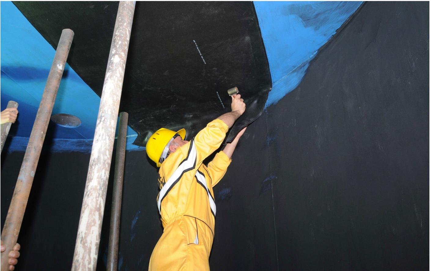
Rubber has long been used as corrosion mitigating lining for metallic surfaces with a broad range of compositions to meet technical requirements for durable resistance to chemicals, abrasive mediums, impact and elevated temperatures.
