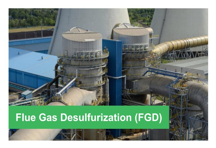
Depending on the scrubbing method, the FGD process may differ; however, there are several pieces of equipment common among all units including steel ducts, absorbers, Gas to Gas Heaters (GGH), Bypass damper, etc. These parts majorly experience highly corrosive/wear conditions due to the combined exposure of corrosive flue gases and solutions, the possibility of abrasion and high temperatures during normal operation and upset conditions.
