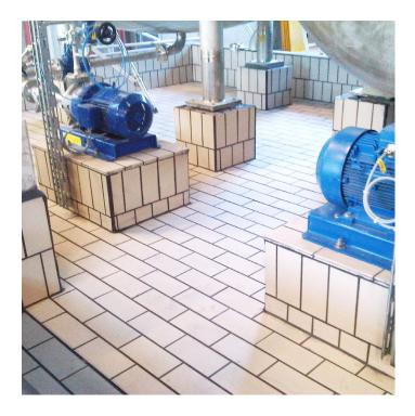
**HEGGEL FU 638** is also remarkably temperature resistant, capable of withstanding temperatures up to 180°C depending on the type of chemical in use.
