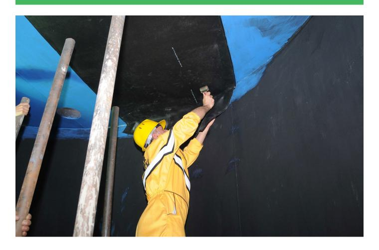
Rubber has long been used as corrosion mitigating lining for metallic surfaces with a broad range of compositions to meet technical requirements for durable resistance to chemicals, abrasive mediums, impact and elevated temperatures.
